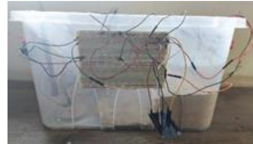
Figure 29 Connection of Sensors to ESP
